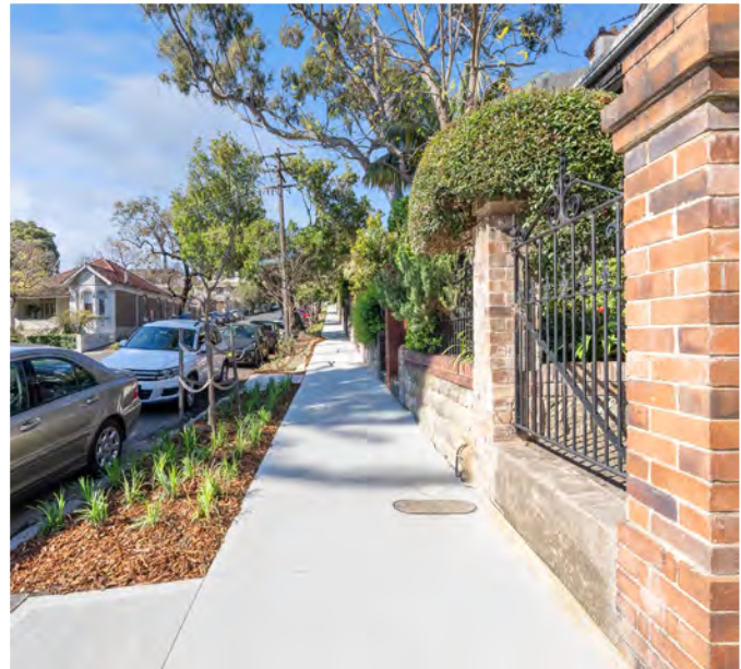
Images: Eglinton Road, Glebe Footway Renewal Works 2021
